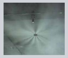
free space at the nozzle outlet to allow a mist to form fully and prevent it hitting a nearby obstacle before it can actually have an effect. With this in mind, WAGNER has tested and developed new types of nozzles with an extremely narrow spray angle which can be directed with precision within the remaining free areas. A space less than 5 cm wide is actually enough to form a full mist.
