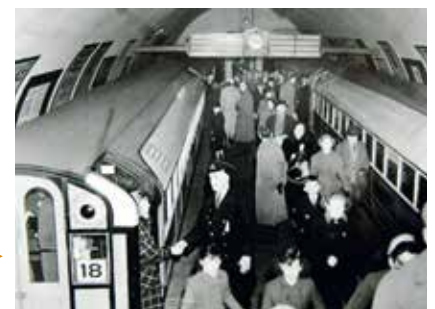
Many stations still look like this: ▶ Narrow tunnels and platforms are not uncommon in Glasgow.
